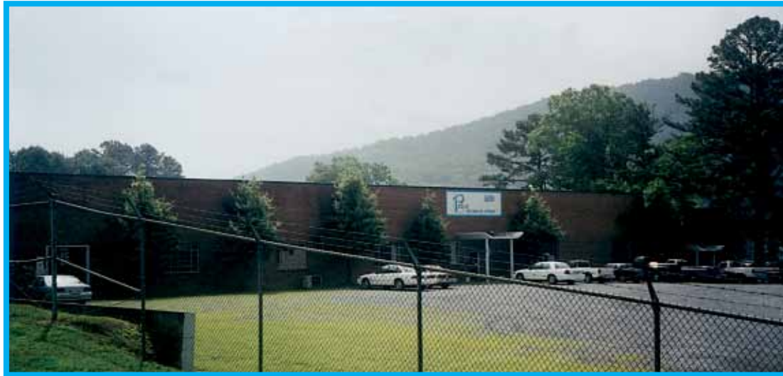
TopFlite Mixing Plant :
